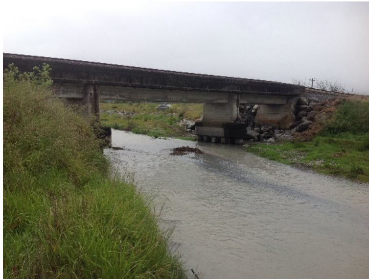
Figure 6.69: Middle Creek Railway Bridge (facing northwest) [-42.3672, 173.6862].
