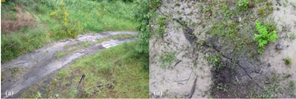
Figure 6.11: Lateral spreading cracks with ejecta near the eastern approach to Waiiau River Bridge [-42.65525, 173.036].
