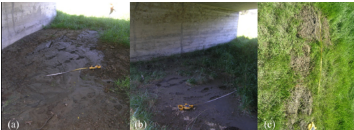
Figure 6.51: Liquefaction ejecta at Needles Creek Bridge site [-41.8217, 174.1370]: (a) Ejecta between piers 1 and 2; (b) Ejecta between piers 3 and 4; (c) Ejecta in free field west of bridge.
